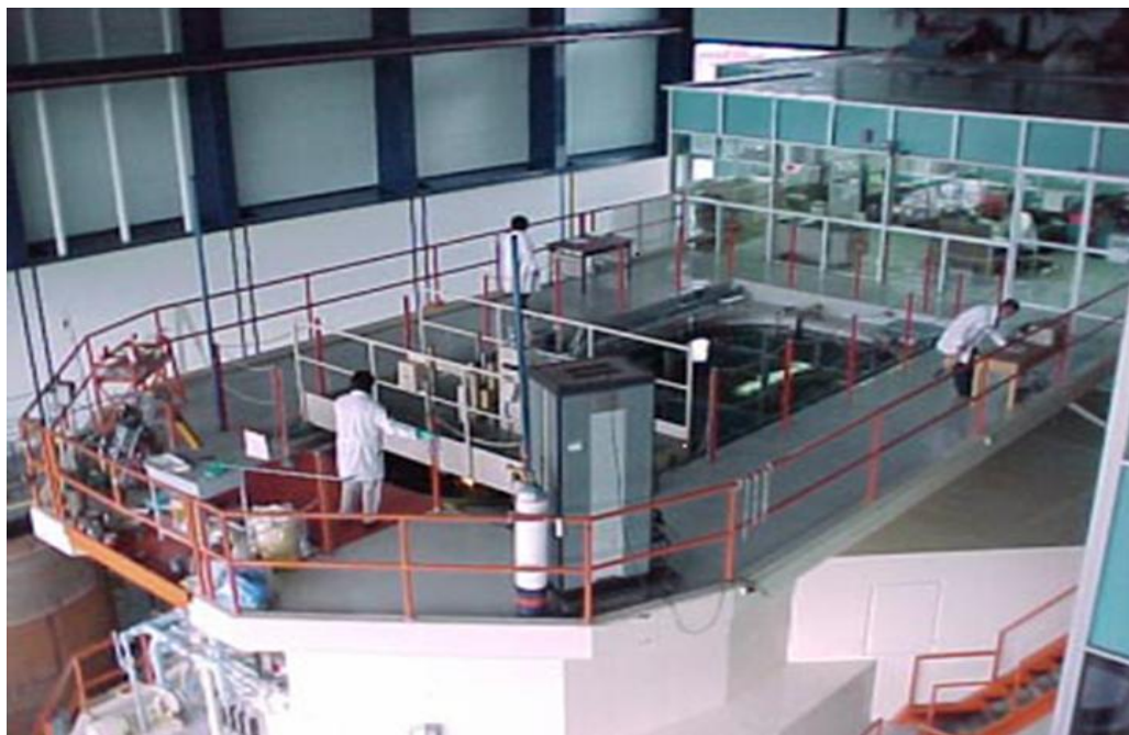
Figura 6 Vista del reactor nuclear TRIGA Mark III (19)
